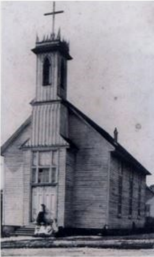
Central's first church structure
